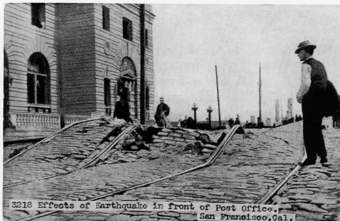
Figure 5. The main post office did survive, although the street and trolley tracks suffered quite a bit of damage.
